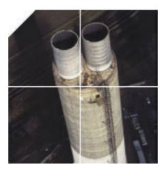
In this case the entire flue can which is supported at the top would experience a very large thermal expansion in the downward direction. If proper arrangement is not provided to compensate this expansion, flue-can would foul with the duct. In addition, the sealing arrangement should also be perfect to prevent leakage of flue gas or fly ash.
