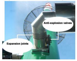
Designing chimneys and stacks to provide the correct amount of natural draught or draft involves a number of design factors, many of which require trial-and-error reiterative methods. One of the key areas for optimization was in Chimney designs – which changed from individual stacks to Multi Flue Chimney.
