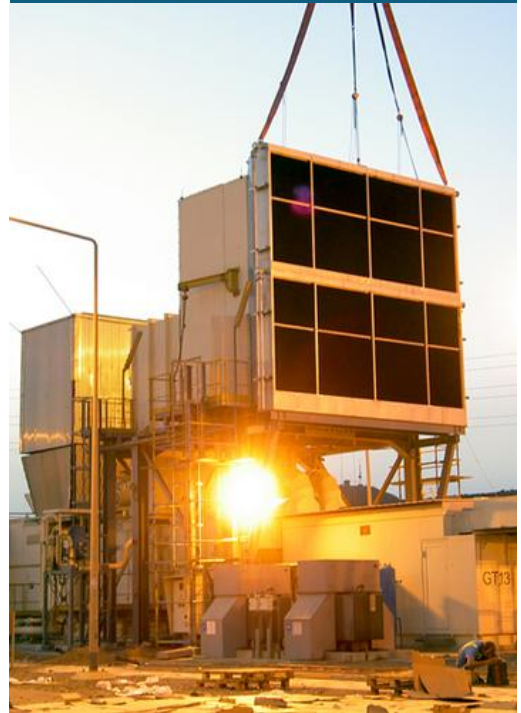
Installation of Munters evaporative air coolers
