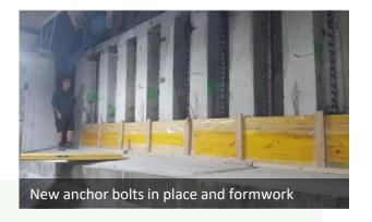
After 24 hours of curing, the first batch of replacement concrete, up to one meter below floor level, was poured. Prior to that a layer of Alphatec 440 epoxy bonding agent was applied to all surfaces to ensure adherence between the existing and new concrete. Then a further grout of Alphatec 800 was poured into the anchor bolt cavities to a level 15 cm below the base frame of the engine.
