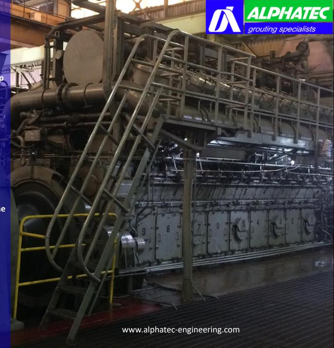
Alphatec-Engineering reports successful completion of repairs to the foundations of a Mitsubishi-MAN diesel engine, type 18V52/55B, at the CUC (Commonwealth Utility Corporation) power plant on the island of Saipan, the largest of the islands that comprise the Commonwealth of the Northern Mariana Islands, located in the middle of the Pacific Ocean
