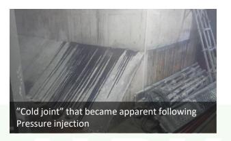
A series of injection holes was drilled alongside the engine and alternator foundation, to a depth of 3.6 m, and Alphatec 342 epoxy resin pressure injected, repairing the "cold joint" that became apparent just above the 45° sloping part of the foundation, as well other separations and stress cracks, raising the effective damping inertia of the foundation.
