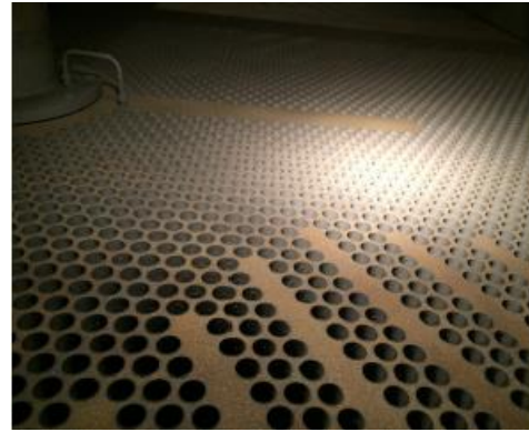
Fig.2b After plastocor® grit blasting
