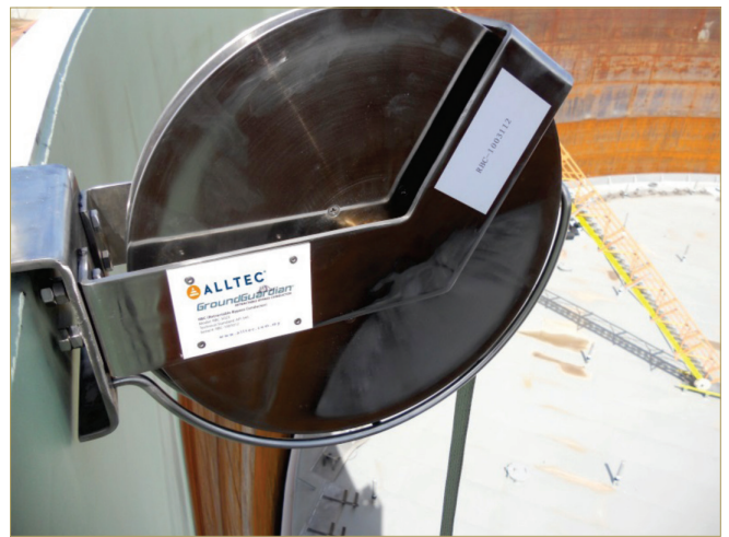
Retractable Bypass conductors installed to address issues related to conductivity on the shunt of a floating roof top tank
