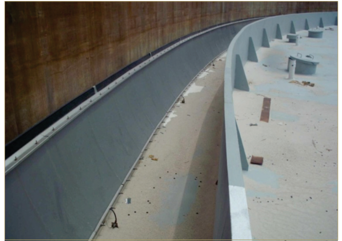
Floating Roof Top Tank - Conductive shunt. Contamination/Residue often builds up to form on the shunt creating two surfaces of non equal potential
