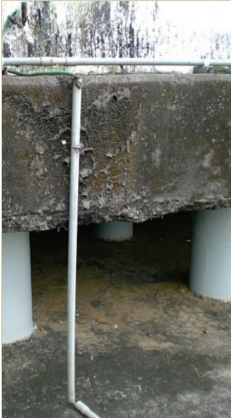
Bonding cable with right angle bends
