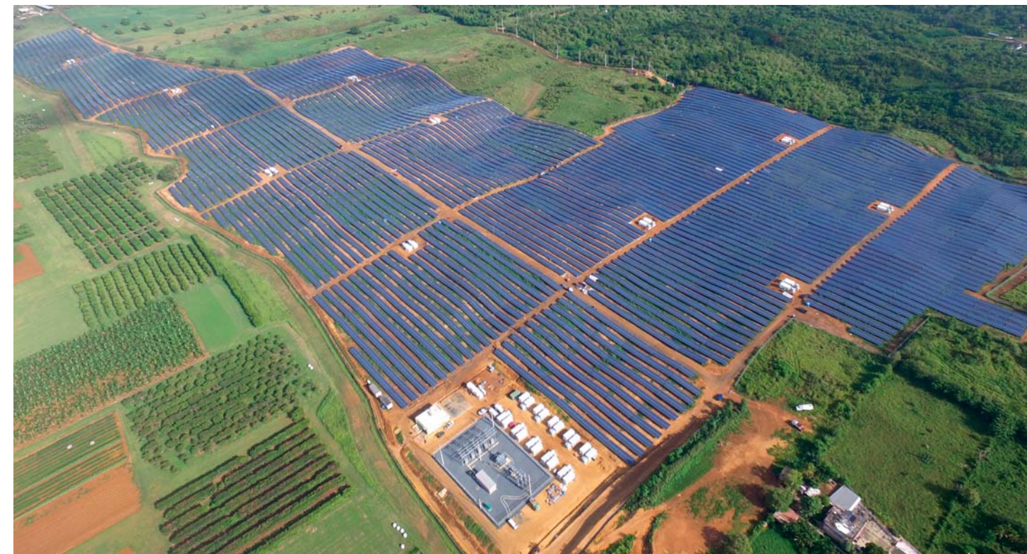
Oriana 57MW PV project in Puerto Rico, including a significant battery installation and HV substation scope
