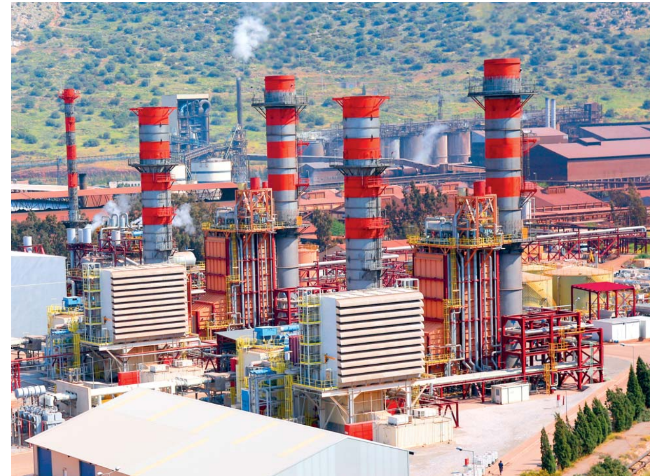
The 320 MW Aluminium of Greece co-generation plant. The plant delivers power to the network and process steam to the alumina plant, which can be seen in the background.
