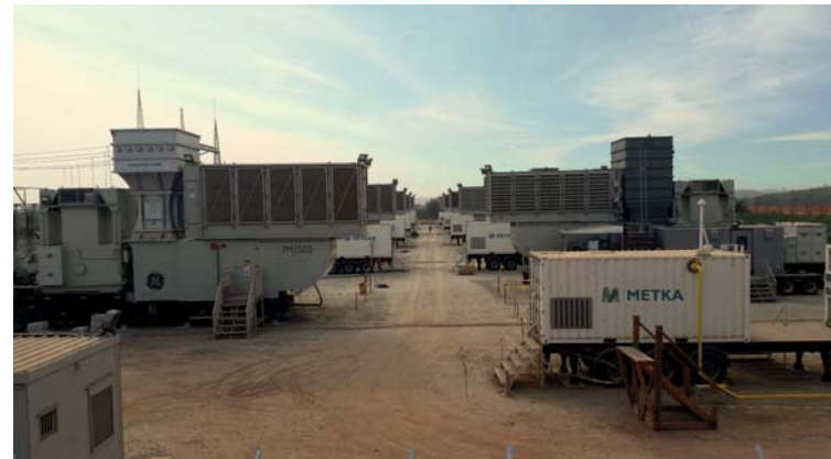
Mobile gas turbine power generating sets installed in Ghana
