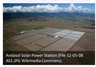
Andasol has a thermal storage system which absorbs part of the heat produced in the solar field during the day. This heat is then stored in a molten salts on two HTF tanks (Heat Transfer Fluid tanks).
