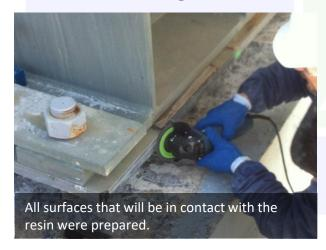
Using pneumatic chippers, we got rid of enough material form underneath the sliding plate to be able to place the first Alphapad® sized D2.
