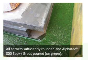
The quantity of material removed was sufficient to ensure a proper levelled surface with healthy concrete, and not enough to change in any way the position of the saddle.
