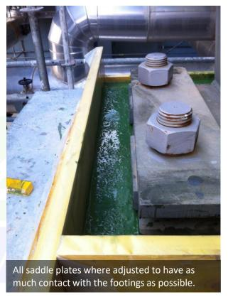
Finishing of all grouted areas was revised to avoid sharp edges and After taking off the pressure on the Alphapads<sup>®</sup>, the whole of the tank weight rested on the epoxy grout.
