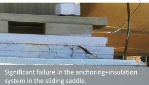
The anchoring+insulation system used for the moving supports is thoroughly deteriorated. The insulation part was designed and built using two different materials, two insolation plates and one cement grout which add up to approximately 110mm in thickness.
