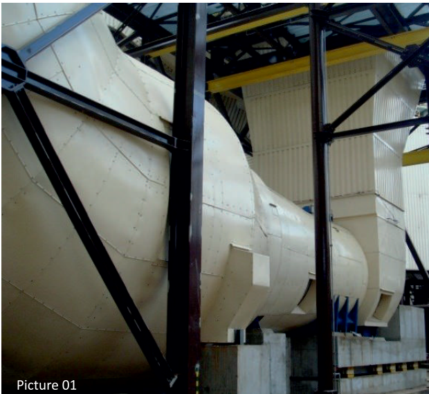
Induced draft fan at site for coal-fired power plant
