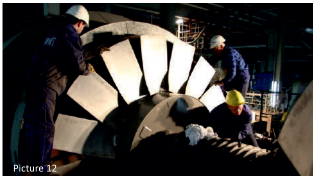
Upgrade of forced draft fan for utility boiler
