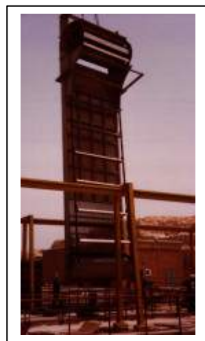
Continuous chain raked bar screen
