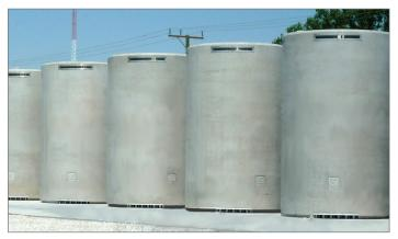
MAGNASTOR incorporates economic, engineering, operations, shielding, and fabrication advantages. **Top photo:** BWR basket. **Middle photo:** Vertical concrete casks. **Bottom photo:** PWR canister and basket.
